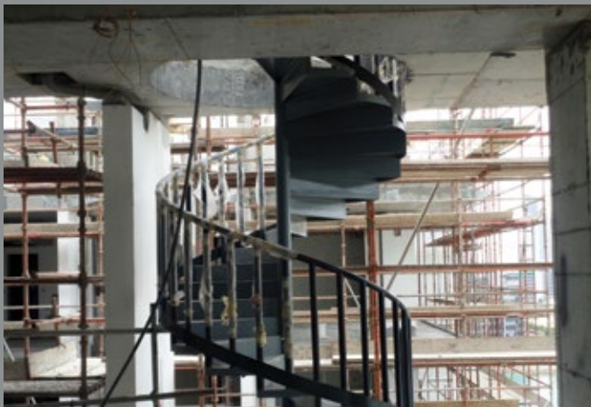
West Side 7th Floor Spiral Staircase
