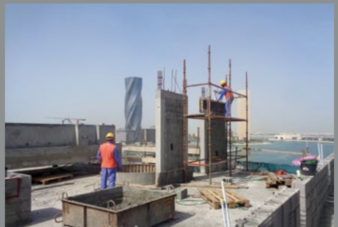
East Side Roof Works Progress
