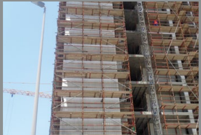
West Side External Painting
