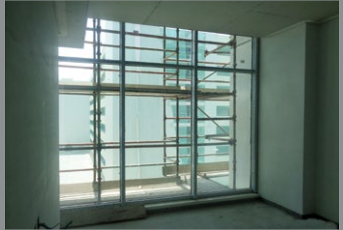
West Side First floor - Glazing work
